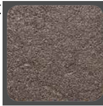
R = Ruggine R = Rust
