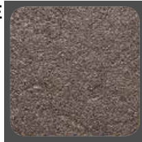
R = Ruggine R = Rust
