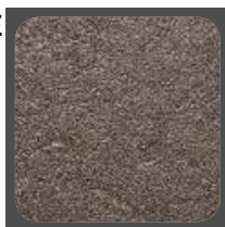
R = Ruggine R = Rust
